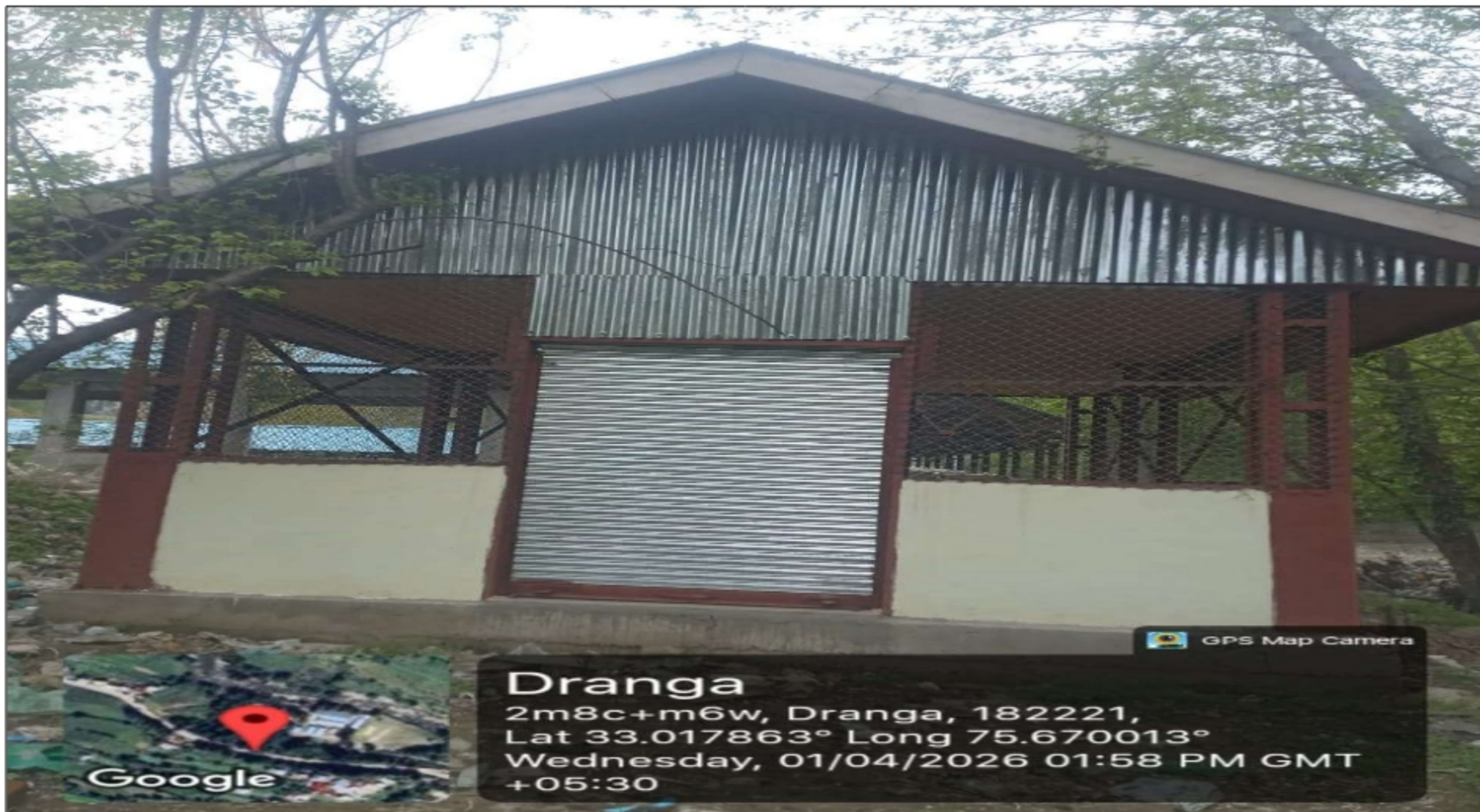
Construction and Demolition Waste Unit at Dranga, Bhaderwah
